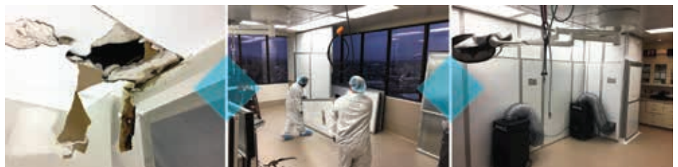
From top: Assessment and remediation of water damage being performed in a temporary STARC containment system. > Remediation and renovation performed with a STARC containment system and negative air.
