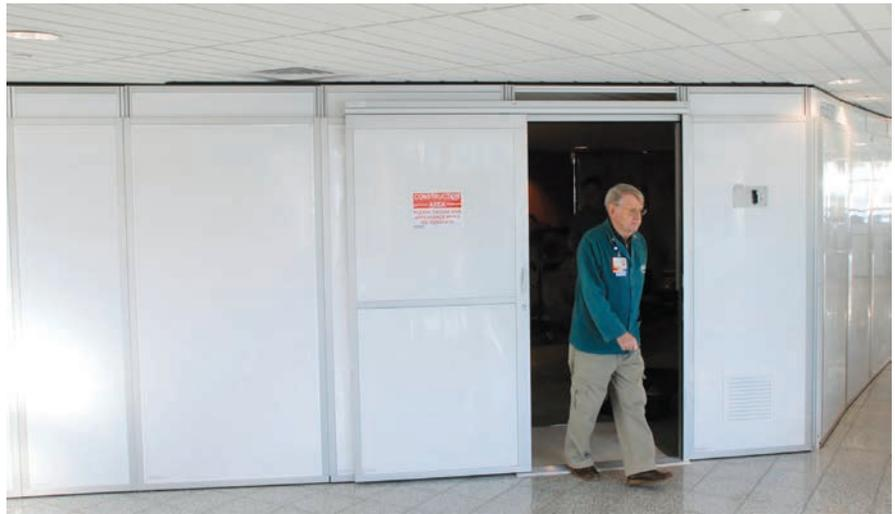
To comply with the ICRA requirement, the renovation required building a 100-foot airtight containment barrier around the construction zone.
